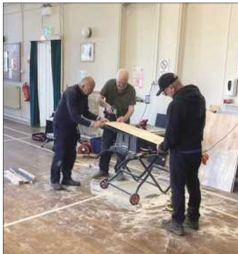
Set-building in progress ... bring on the tea and biscuits!
